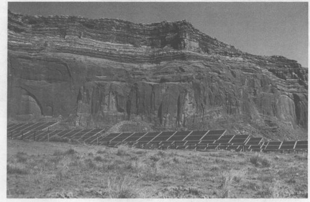
ROWS of solar photovoltaic panels line the shore near the Dangling Rope Marina on the remote north shore of Lake Powell in southern Utah. The photovoltaic system began operating this summer, replacing a dieselpowered generator that was costly to operate, noisy, and polluting. Sandia tested the photovoltaic system's power converter for six weeks.
